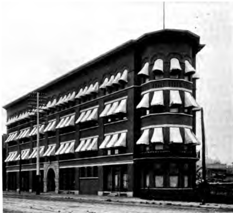
SOUTHERN EXPRESS COMPANY'S BUILDING.
